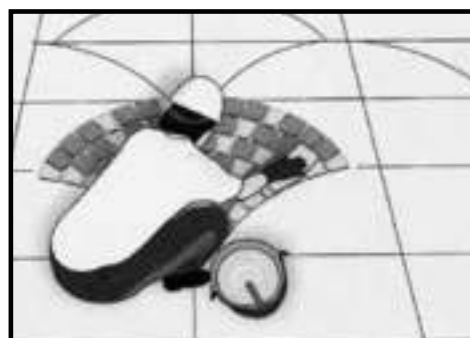
6. Use sponge with water to clean adhesive and leave at least 1 day then grouting
