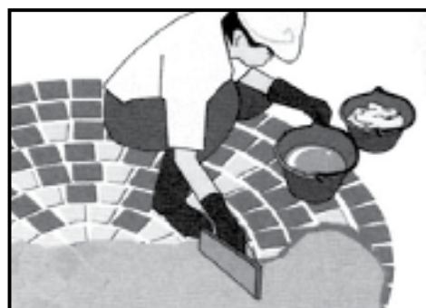
7. Pour water on the tile and use wooden trowel with Kbond Sanded Grout for grouting
