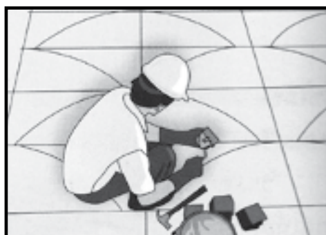
3. Apply adhesive at the back of tile
