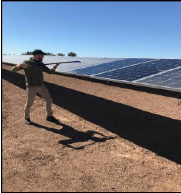
On site in El Centro, California
