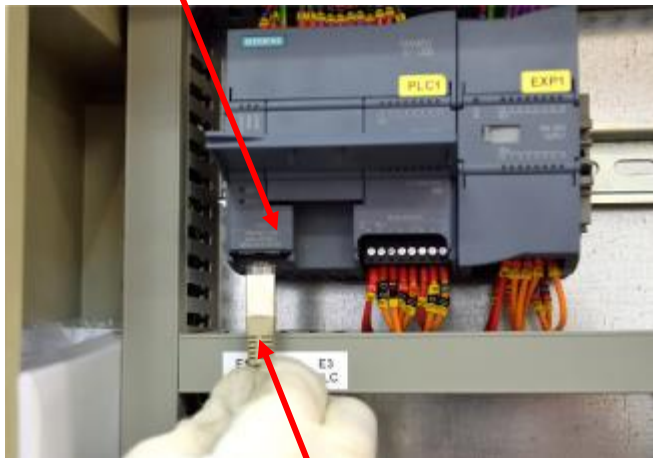
Communication Connection terminal
