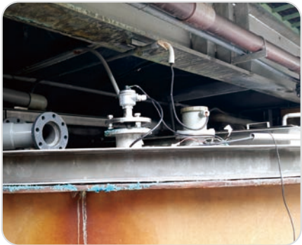
Copper sulfate storage tank
