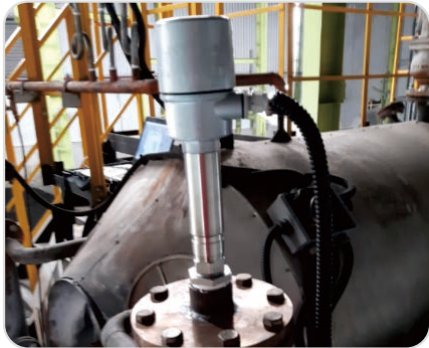
High temperature boiler
