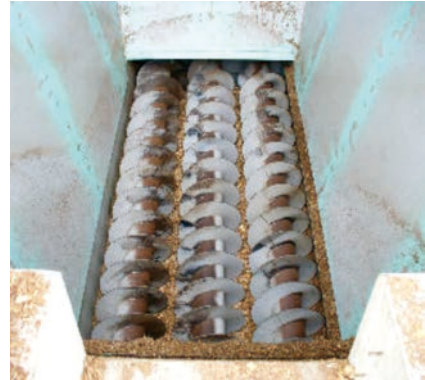
Mounting in discharge screw (wood-fired power plant)
