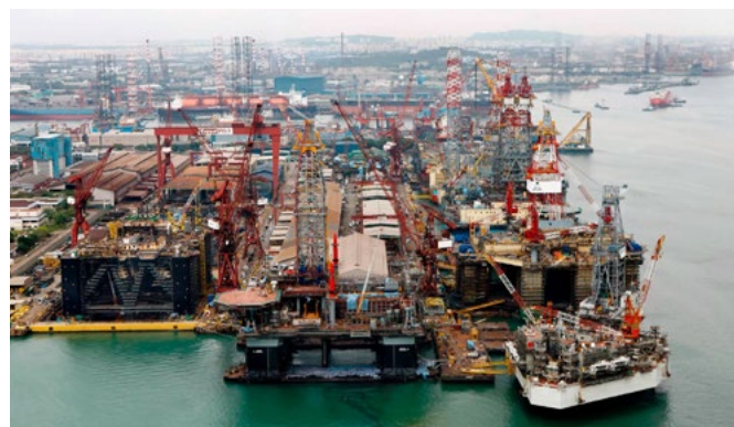
Giàn khoan Drilling oil rig
